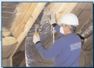
Between Roof Joist
