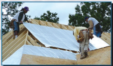
Beneath Roof Deck
