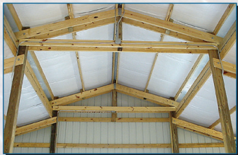
Wood Purlin on Wood Truss
