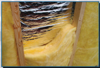
Behind Fiberglass Batts in Walls to Reduce Cooling Costs
